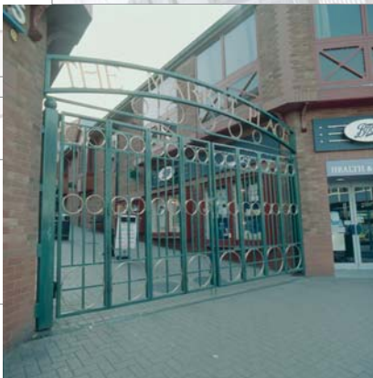
4. Custom designed ornamental gate
