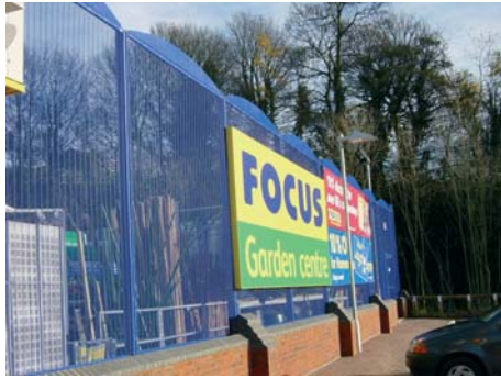
7. Bespoke welded mesh fencing
