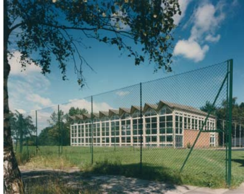
2. Chainlink on steel posts
