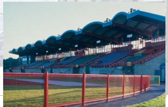
12. Running track railing and gates with mesh panel infill
